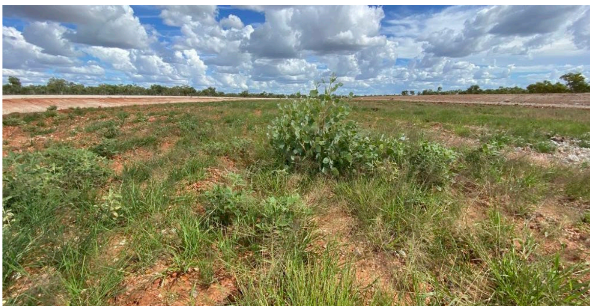
Figure 6. Revegetation works at Lady Annie operations
