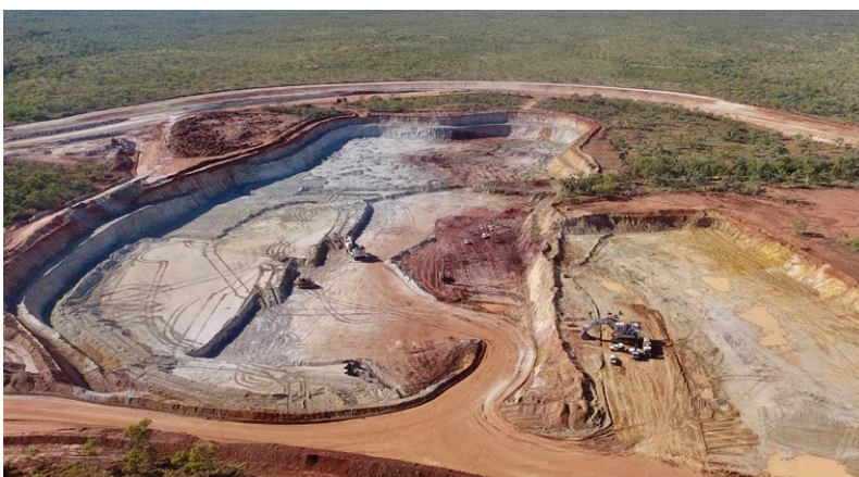
Figure 1. Aerial shot above Anthill East Pit
