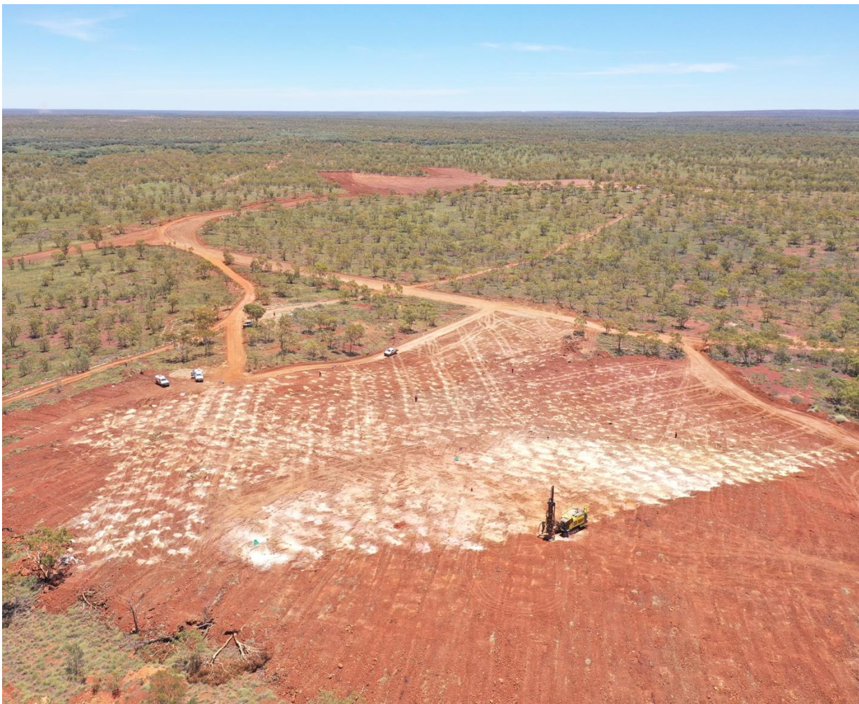
Figure 2. Anthill east pit area showing drilled area for first shot. Haul roads have been marked out for construction.
