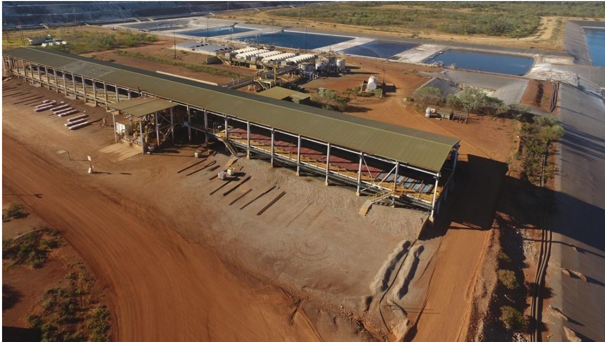
Figure 1. Mt Kelly electrowinning tank house and copper cathodes in foreground, solvent extraction circuit in the background with raffinate ponds.
